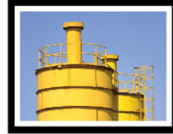
SEWAGE TREATMENT PLANT
