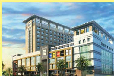
Raksha Business Center On-going Project
