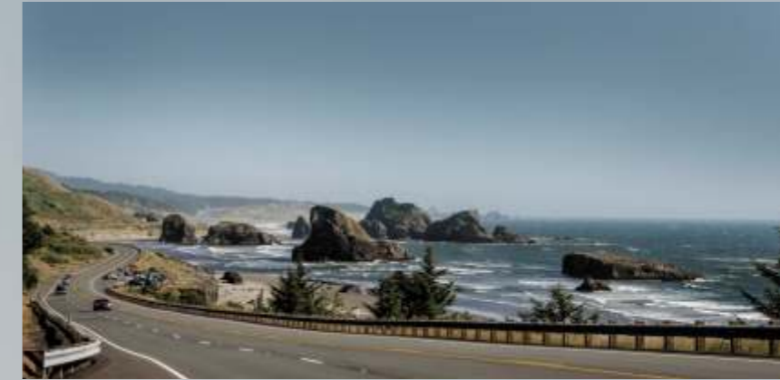
Entry Point of Proposed Coastal Road from Malad (w) to Bandra-Worli Sea Link (2.5 Kms)
