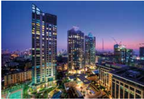
Harbourside, Hong Kong
