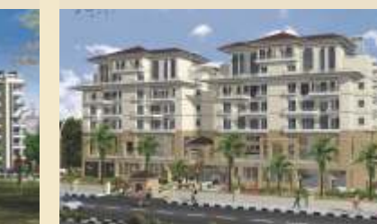
FOUNTAIN SQUARE MALVIYA NAGAR, JAIPUR
