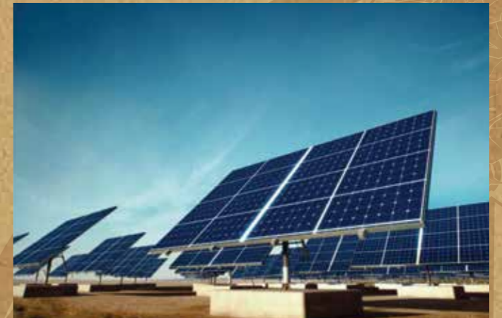
▲ Solar Power for Common Areas ▼
