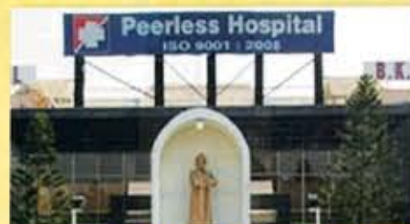
PEERLESS HOSPITAL : 4.0 KM.
