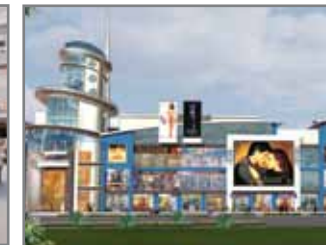
Singapore Mall cum Multiplex Lucknow
