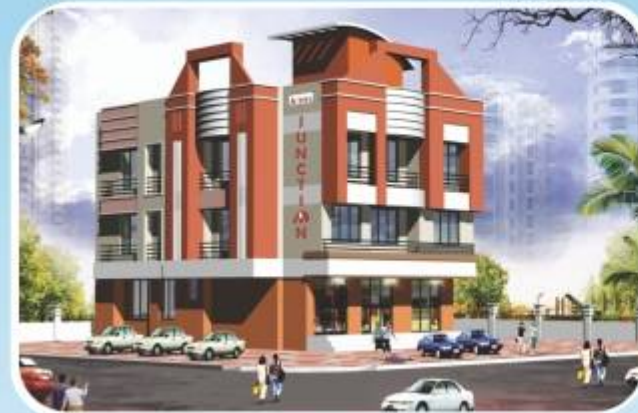
Aims Junction - Bhayander (East), Mumbai
