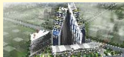
Splendor Epitome-Work 'n' Stay, Sector 62, Gurgaon CONSTRUCTION IN FULL SWING
