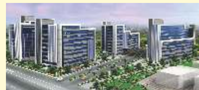
Splendor Spectrum One-Commercial, Sector 58, Gurgaon CONSTRUCTION IN FULL SWING
