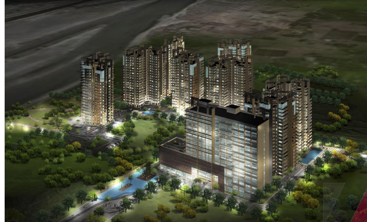
OLYMPIA OPALINE Chennai modern integrated self sufficient township 17-acres 1000 Apartments
