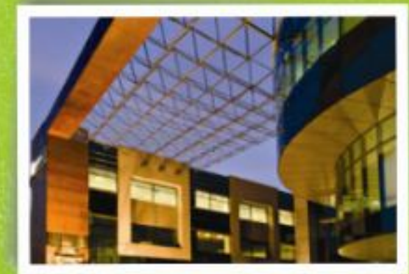
PATNI KNOWLEDGE CENTER, NOIDA (BLOCK B) GOLD RATED LEED CERTIFIED GREEN BUILDING - 2011
