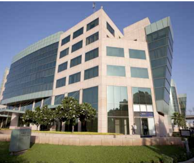
◀ Unitech Business Park-Gurgaon
