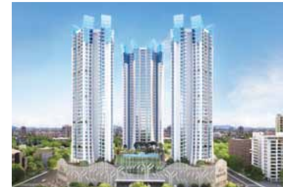
EKTA TRIPOLIS 36 storey residential tower with 2, 3 & 4 BHK luxury apartments at Goregaon (W).
